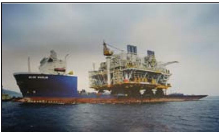
The Compression, Utilities and Quarters platform for Bayu-Undan was built in South Korea and delivered to the Timor Sea in June 2003.
