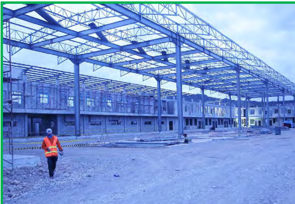
Suai airport under construction – Helicopters hangar
