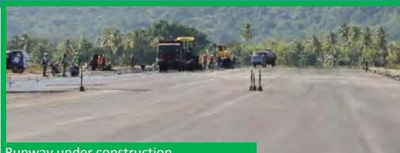
Runway under construction
