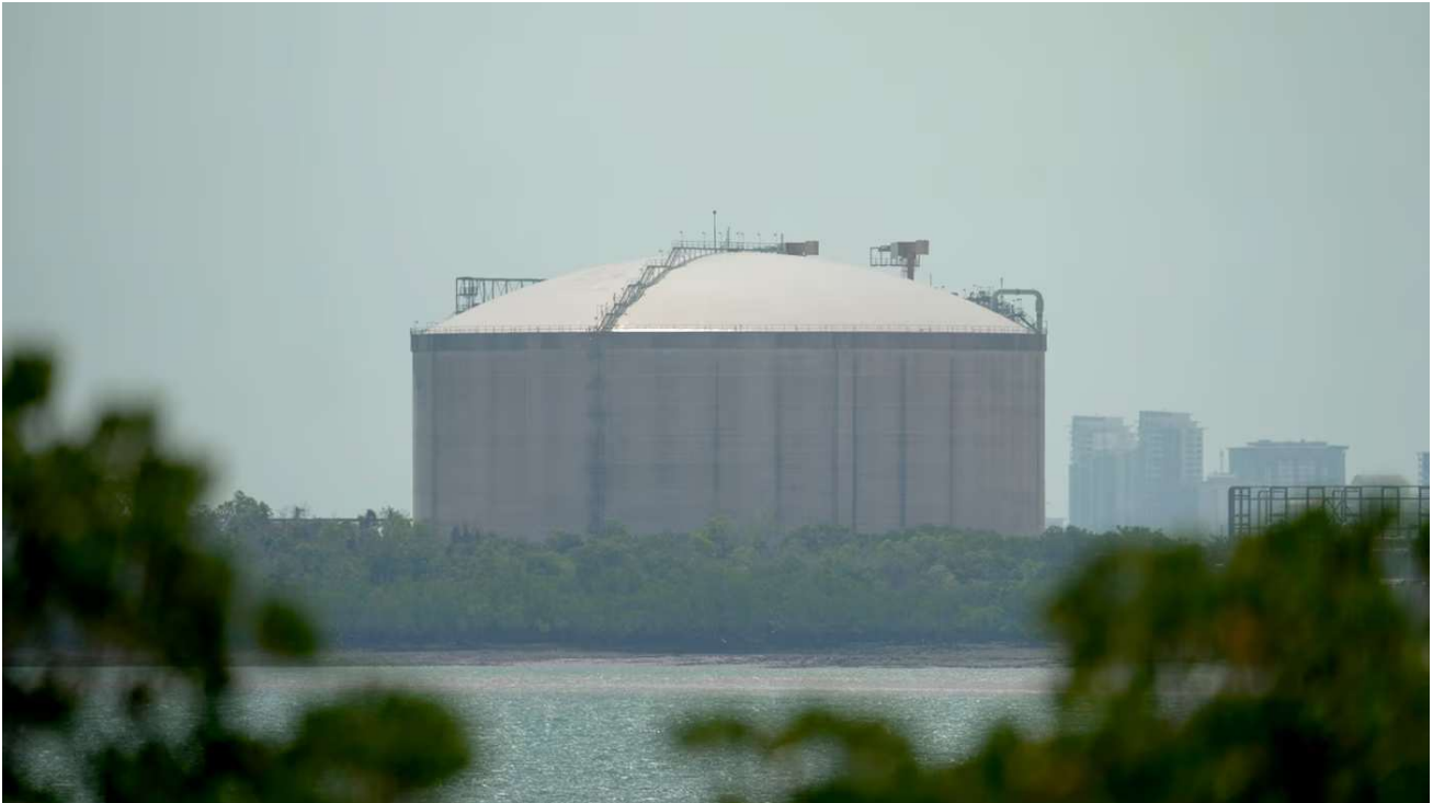
The LNG tank is about 7 kilometres from Darwin. (ABC News: Tristan Hooft )
