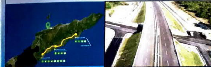
Photo of South Coast project and the first stage of the highway.
