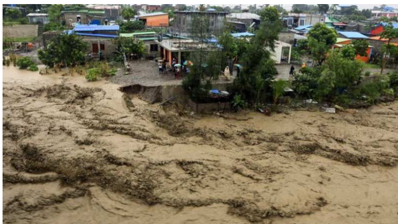
Figure 1. Destroyed houses alongside the Comoro River flooding in Dili, 4 April 2021
