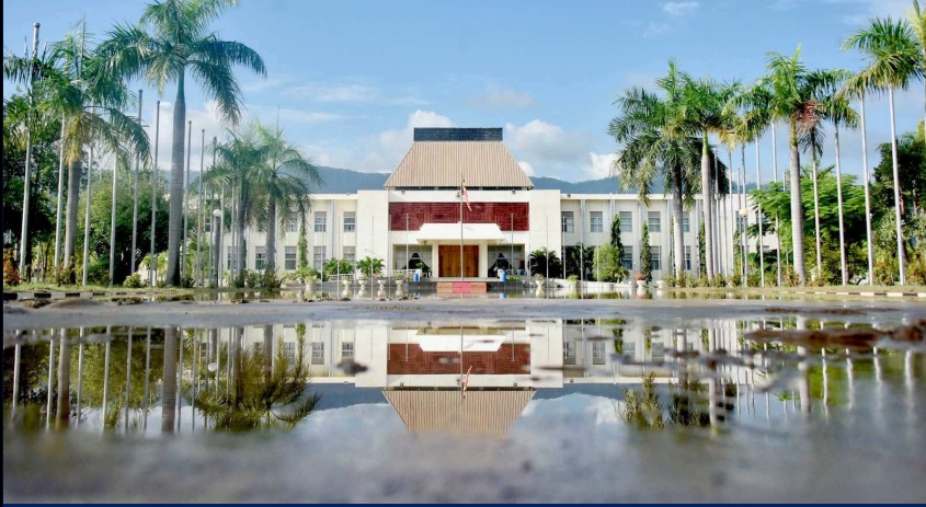
Presidential Palace after April 2021 flooding
