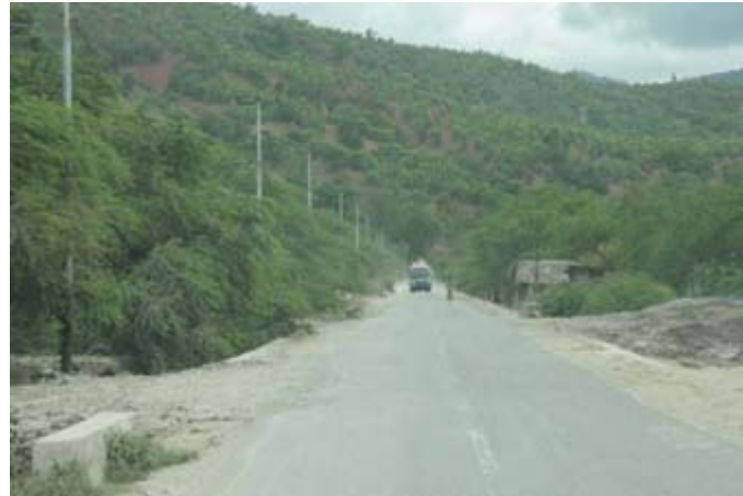
Plate 9 A03-01 route in Tibar traversing the mudflat. Vegetation alongside the road is mostly Prosopis pallida , a mesquite tree commonly found in coastal areas
