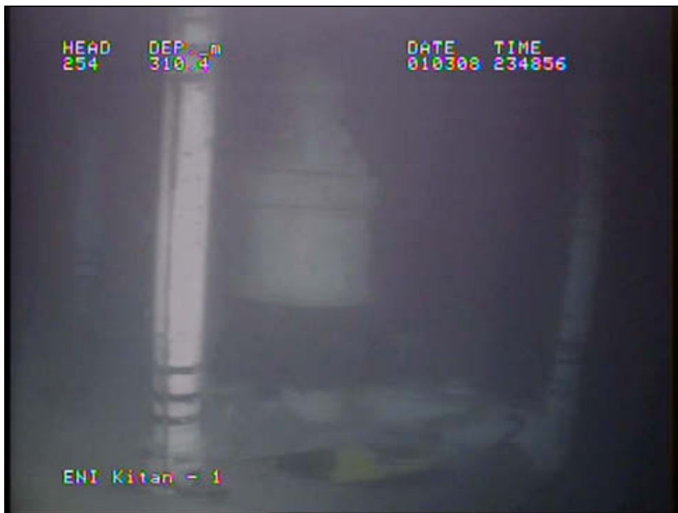
Figure 3.6: Well head clearly visible from several metres away
