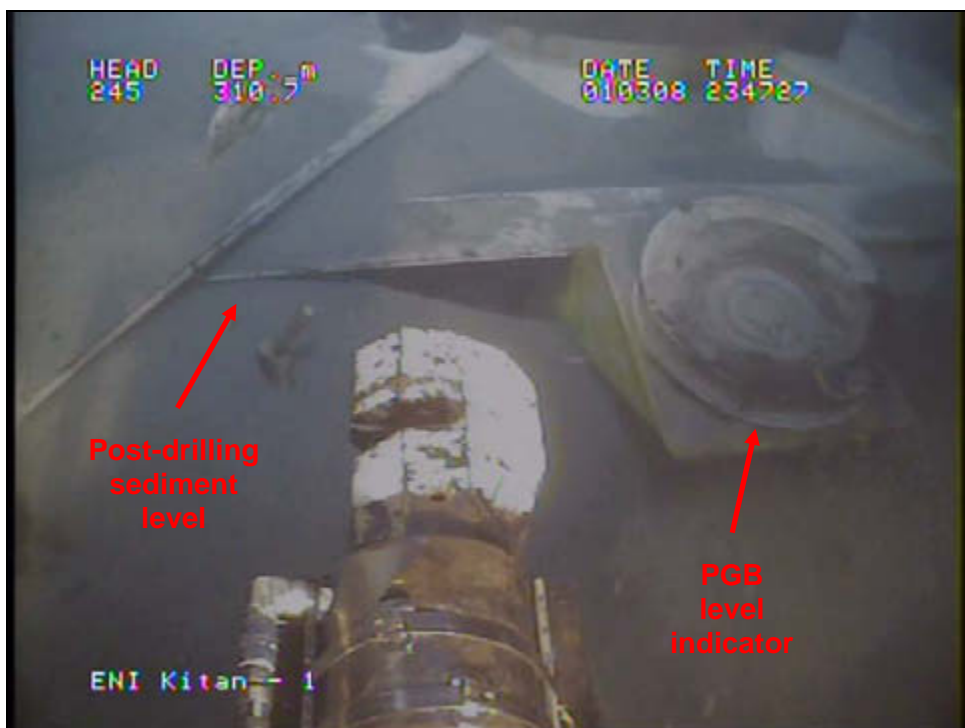
Figure 3.2: View of PGB (upper background) showing sediments at or slightly covering its base
