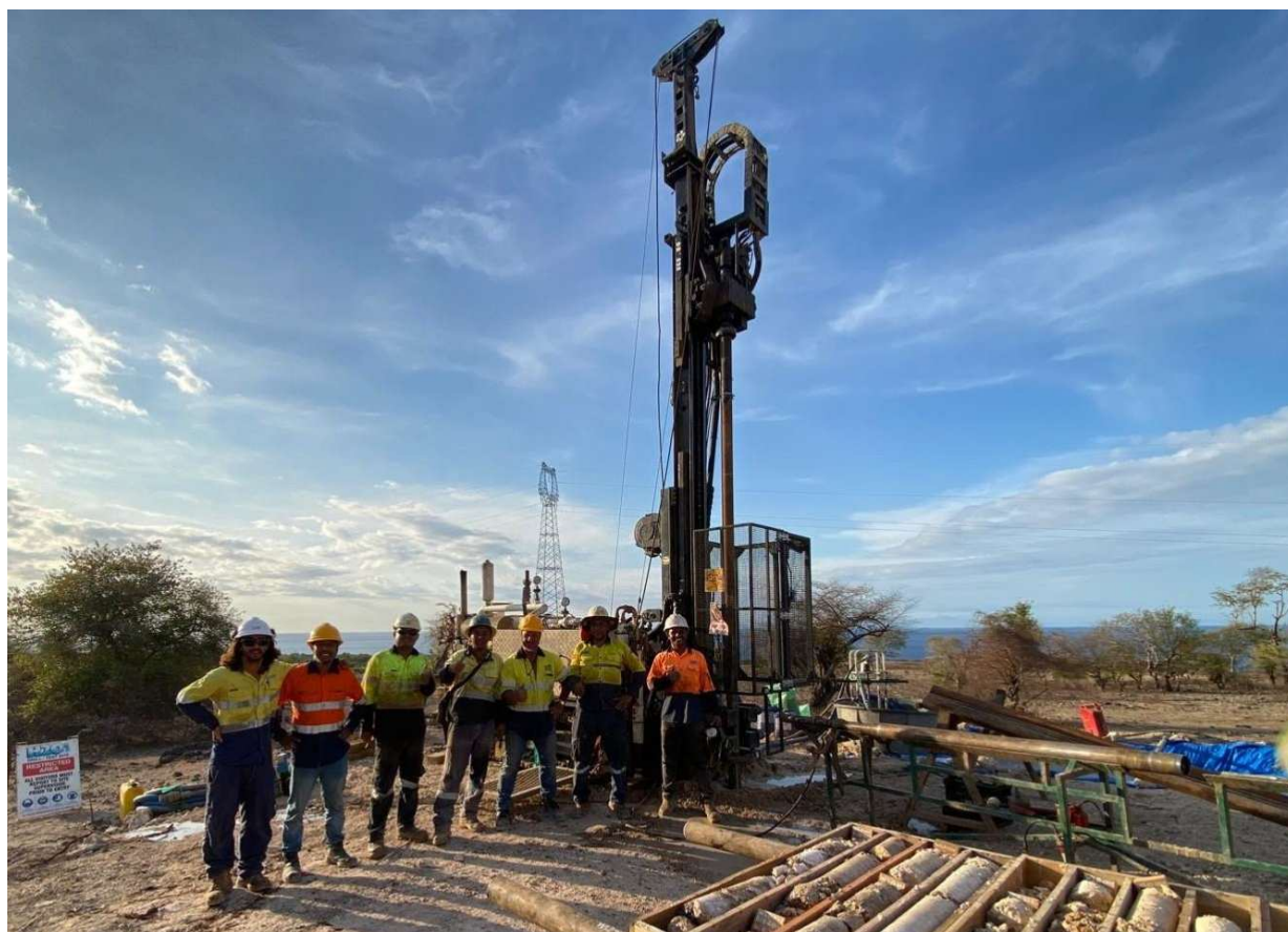
Estrella drills the first hole in the Werumata limestone project in Timor Leste, formally East Timor. Credit: File
