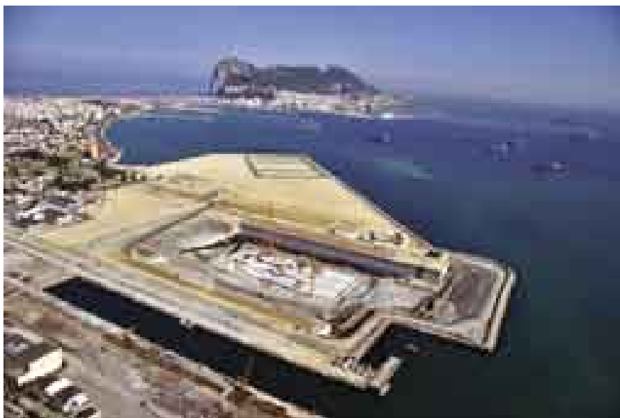
The Campamento construction site at Algeciras, Spain. This -20 m deep casting basin will be used for construction of the concrete Gravity Based Structure. The LNG tanks and topside regasification facilities will integrate with the concrete structure prior to flooding the basin and towing the completed structure to the Adriatic
