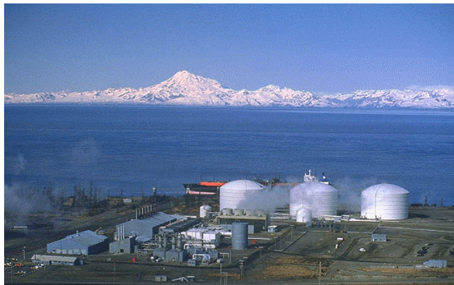
Figure 5. LNG Liquefaction Facility in Kenai, Alaska
