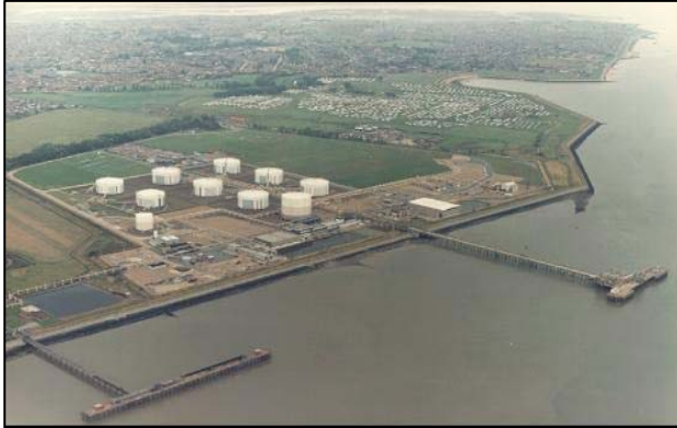
British Gas Canvey Island LNG Terminal, A World First. Source: BG
