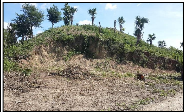
Borrow Pit 6 in Branch 4 Access Side
