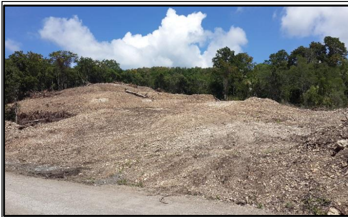
Borrow Pit 4 in Branch 3, Access Side
