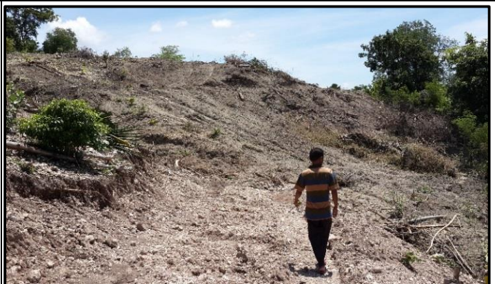
Borrow Pit 2 Sta.14+900 in Branch 2
