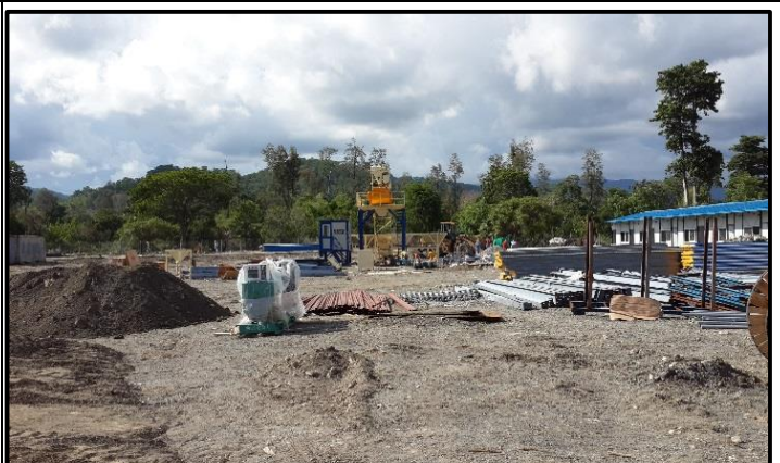
Branch 3 Concrete Mixing Plant and Yard
