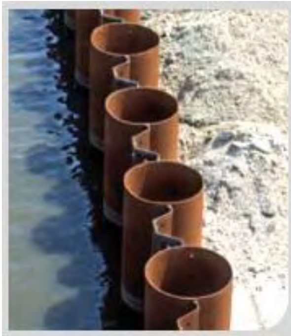
Figure 6-10: Example of a pile wall
