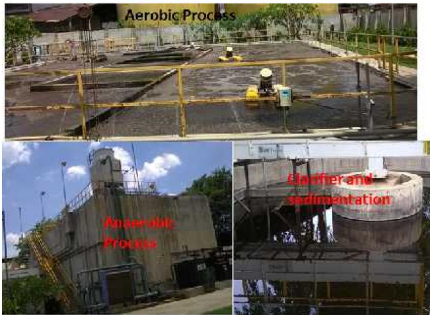
Figure 4.23 Typical Aerobic Treatment of Wastewater Effluent in the Brewing Process
