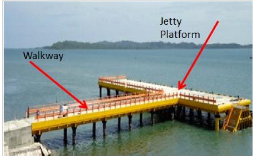
Figure 2.6 Typical Support Structure of Jetty or Above Water Platform
