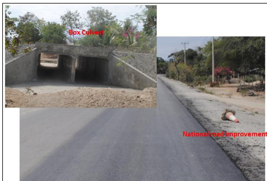
Figure 5.3 Box Culvert Placed under the National Road
